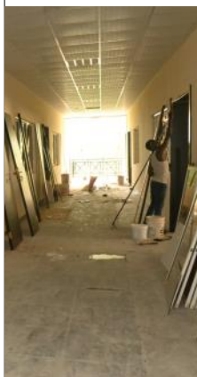
Fixing of windows and doors
