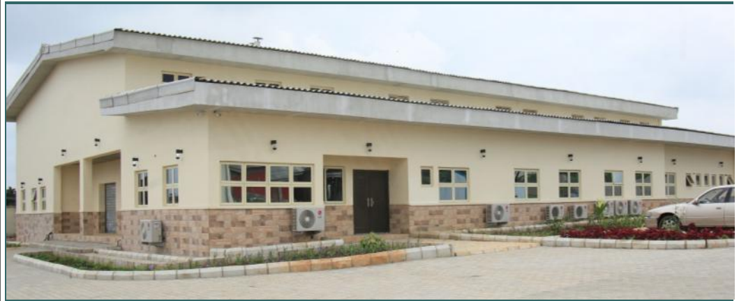
An ultra-modern Babcock Bakery edifice
